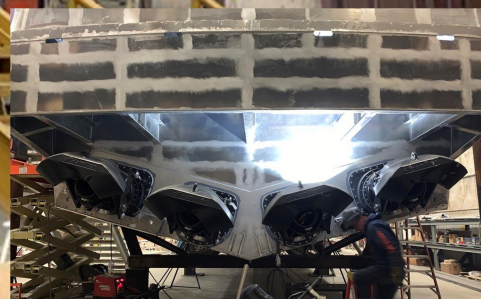
Waterjets mounted on the stern of William Richard Photos courtesy of Shepler's
