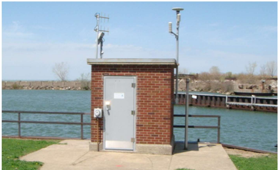
Pictured above is the water level gauge station at Cleveland, OH. Stations like this one are located all across the Great Lakes to monitor water levels.
