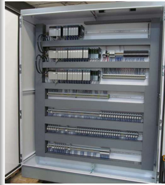
Inside a typical PLC/IO Controller Box. Photo by Randy Barr
