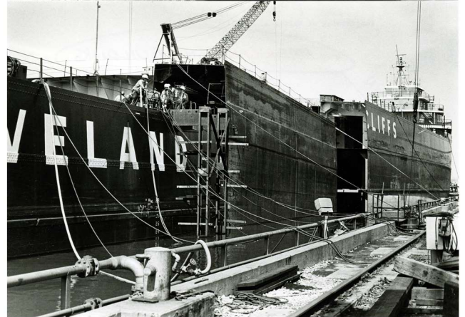
The new midbody for the Walter A. Sterling (now Lee A. Tregurtha ) is floated into place in the drydock at American Shipbuilding in Lorain, OH, July 1976. Press photos, Roger LeLievre Collection
