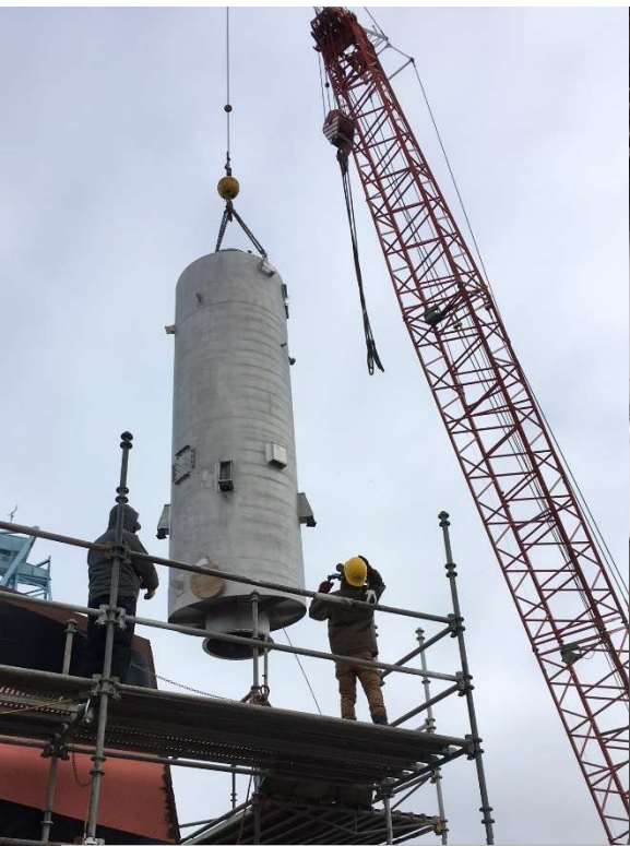
(Left): Lowering one of the main scrubber units into place onboard the Mesabi Miner , 2017. (Right): Scrubber units set in place inside the stack onboard the Mesabi Miner , 2017. Photos courtesy of Interlake Steamship Co.
